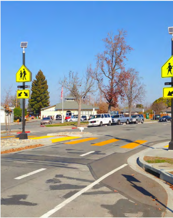
Example: Rectangular Rapid Flashing Beacon
