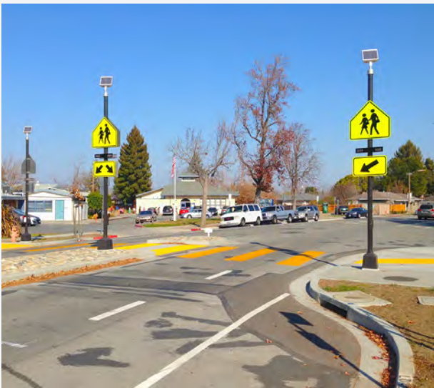
Example: Rectangular Rapid Flashing Beacon
